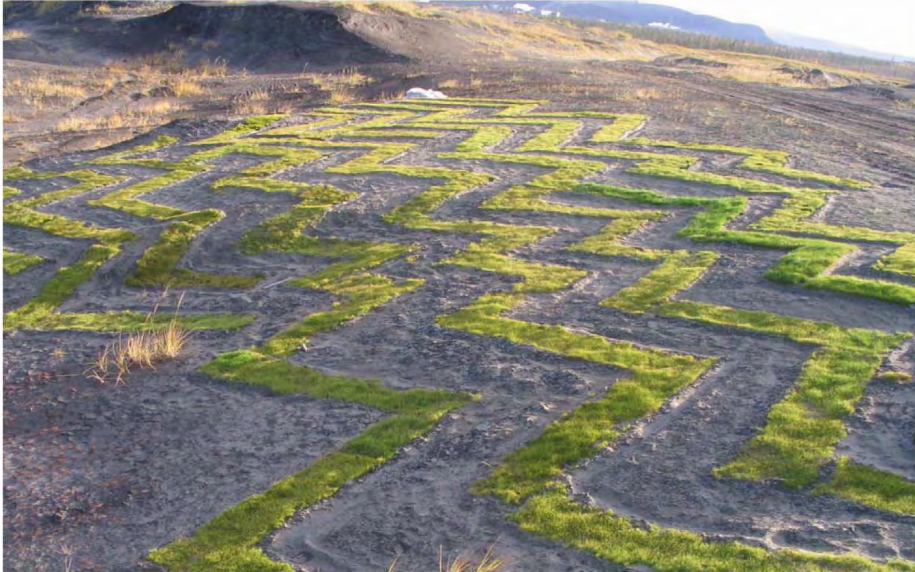
“Chevron-packing” of VIPON-substrate on waste-storage of Apatite-company
